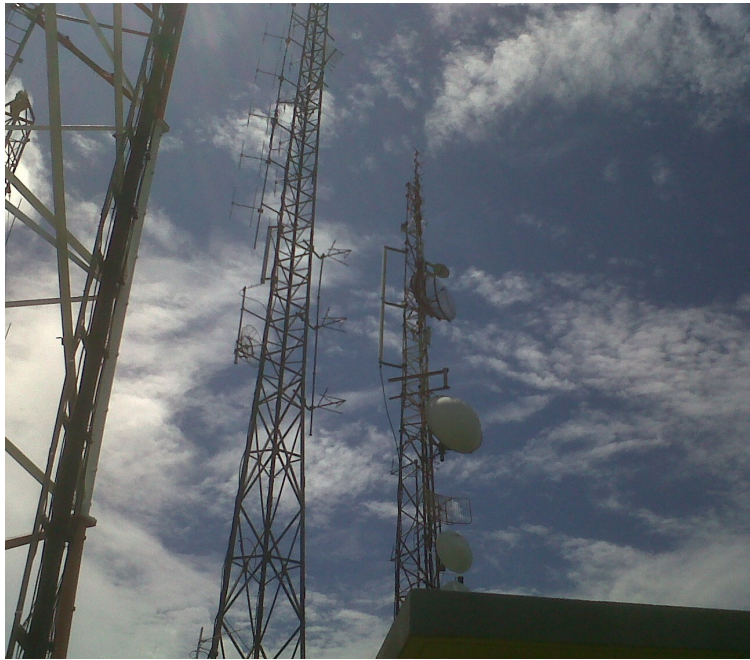
Towers constructed in Trinidad and Tobago
